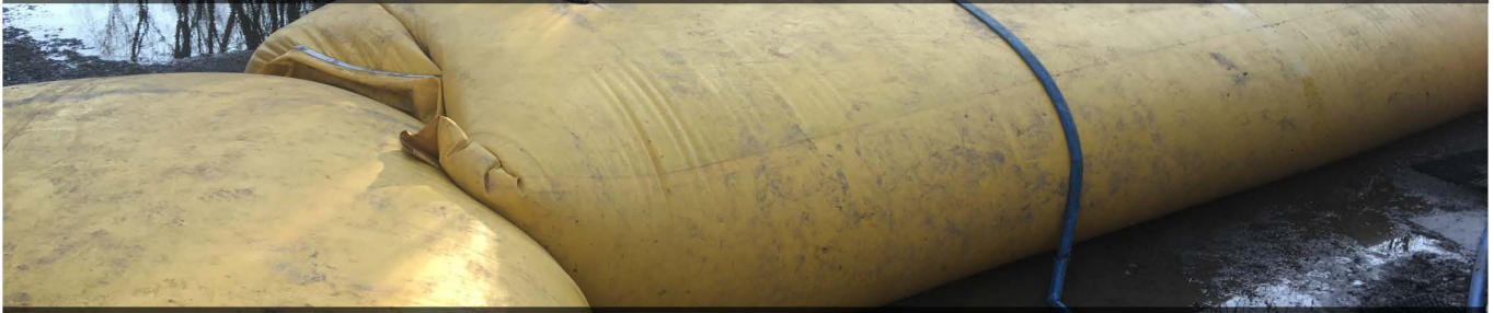
Shekinah's WaterBloc dam in action, shortly after the flood waters had receded. Water rose to within an inch of flooding the chalet.
